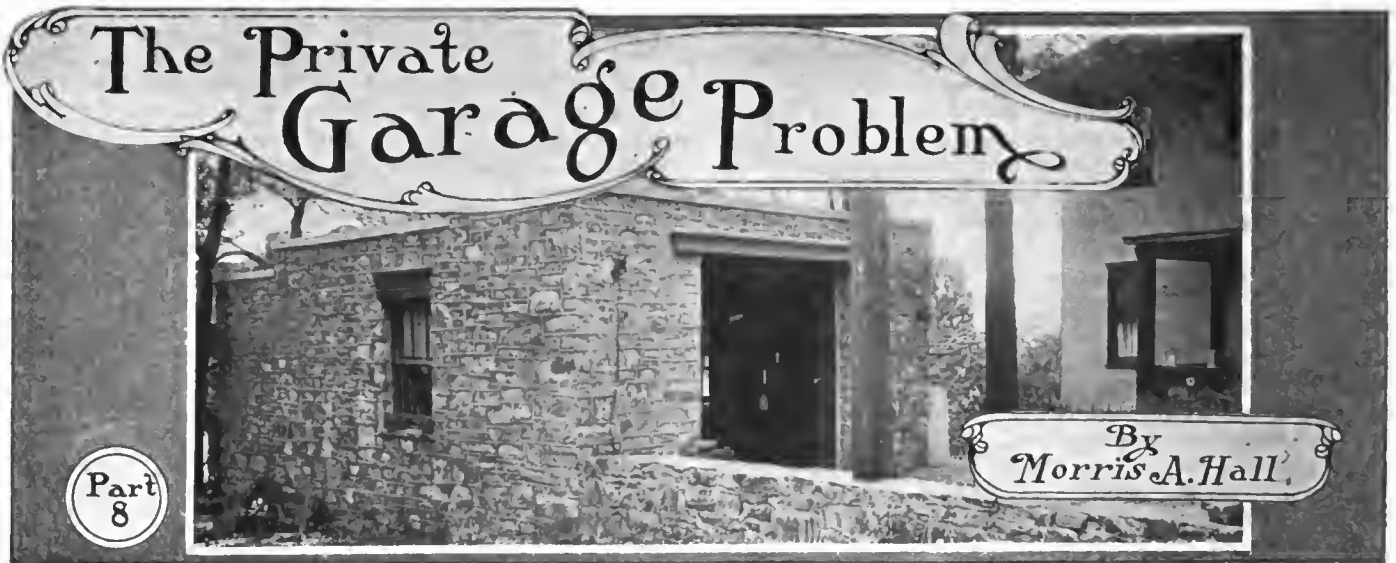
One-Car Garage of Squared Field Stone, Which Appears Well and is Very Well Arranged Inside
